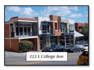
commercial and office spaces on the first and second floors. The exterior improvements consisted new windows and doors, new steel balconies on the second, exterior steel stair towers, and painting. The owner also performed extensive interior renovations and updates for the retail and office spaces. The low bid for qualified exterior façade improvements was \$248,730, for
